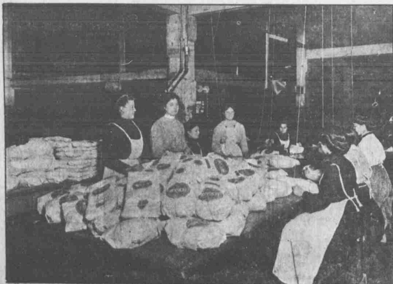
THE COLD STORAGE WAREHOUSE AT ARMOUR'S.
