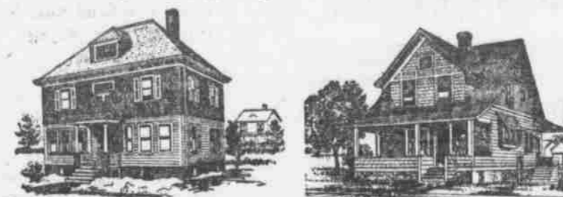
A No. 17-S-W IDEAL Boiler and 300 ft. of 38-in. AMERICAN Radiators, costing the owner $145, were used to Hot-Water heat this cottage. A No. 1-2-W IDEAL Boiler and 400 ft. of 38-in. AMERICAN Radiators, costing the owner $200, were used to Hot-Water heat this cottage.
