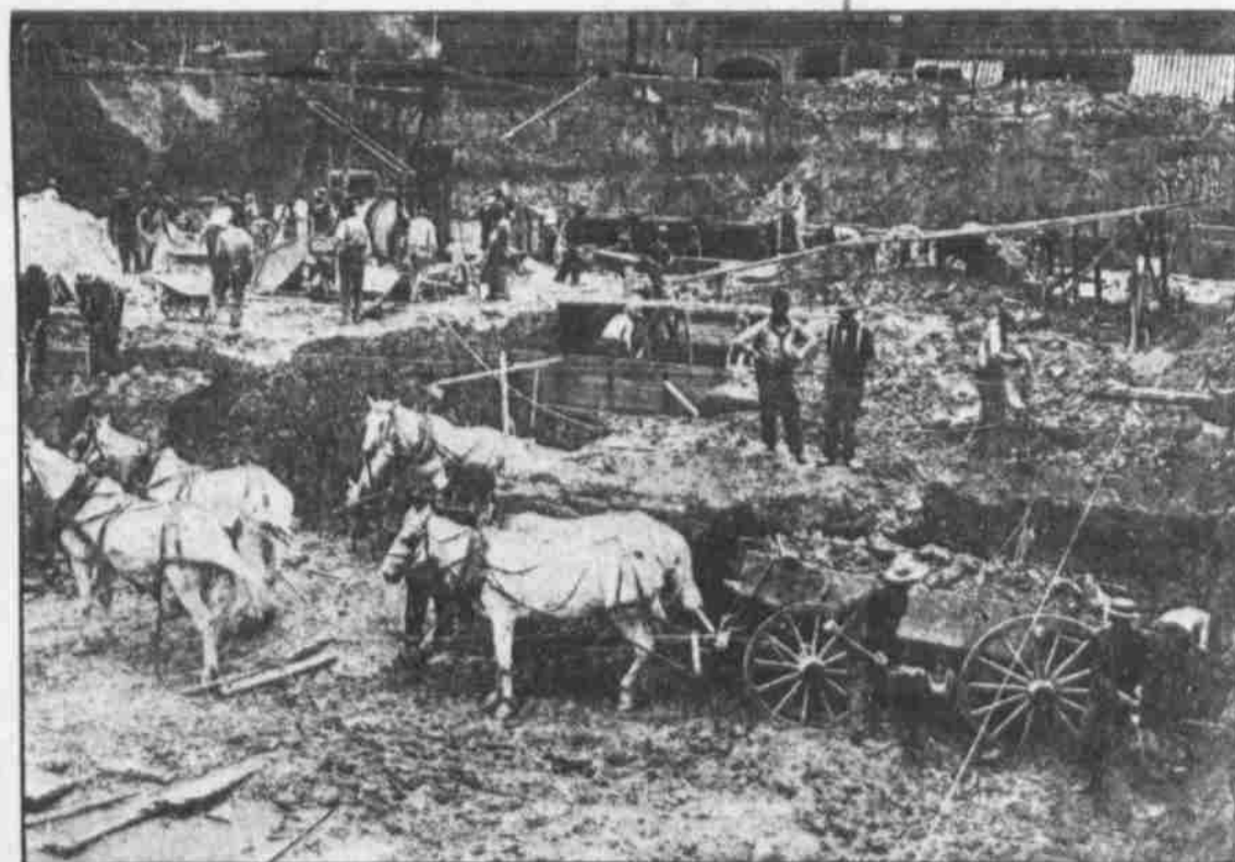
EXCAVATING FOR FOUNDATION PIERS FOR NEW BRANDEIS THEATER.
