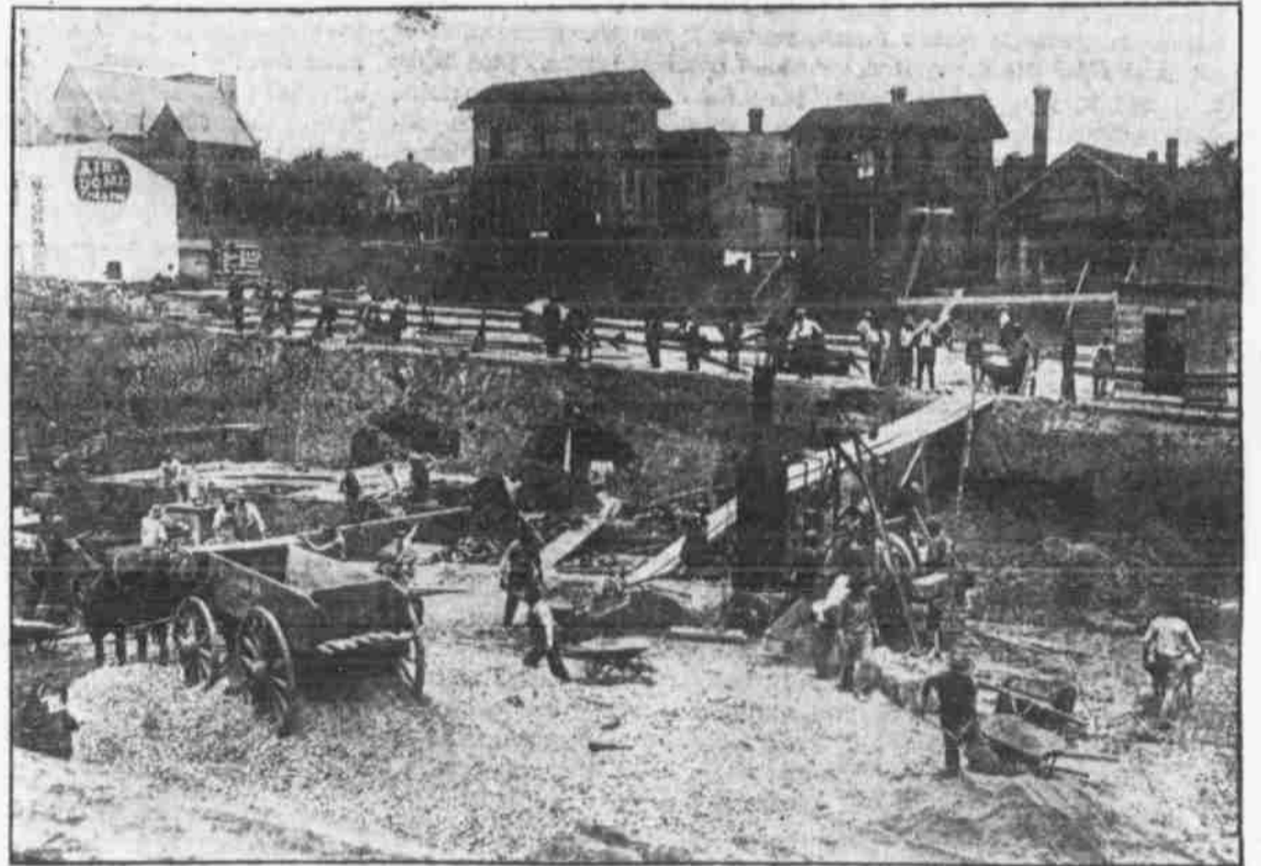
CONCRETE MIXER AT WORK ON NEW BRANDEIS THEATER.
