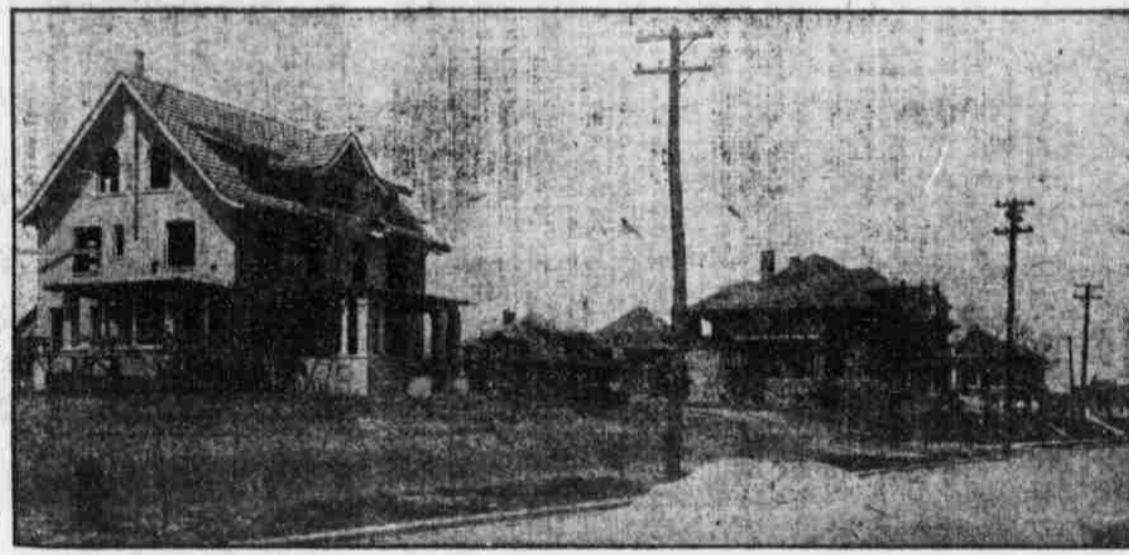
THIRTY-EIGHTH STREET, CASS TO CALIFORNIA. THESE HANDSOME RESIDENCES HAVE ALL BEEN BUILT THIS YEAR.
