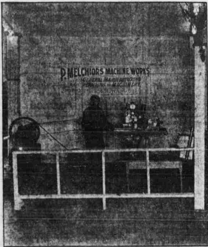
PETER MELCHOIR'S MILLING MACHINE CUTTING GEARS WHILE YOU WAIT.
