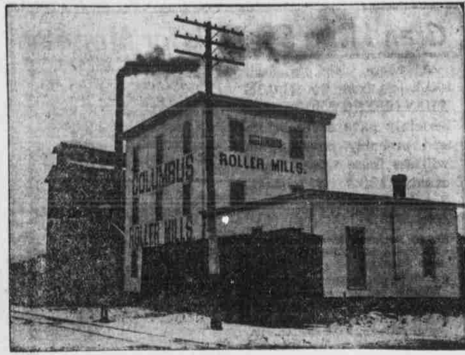
ONE OF PLATTE COUNTY'S FLOURING MILLS.
