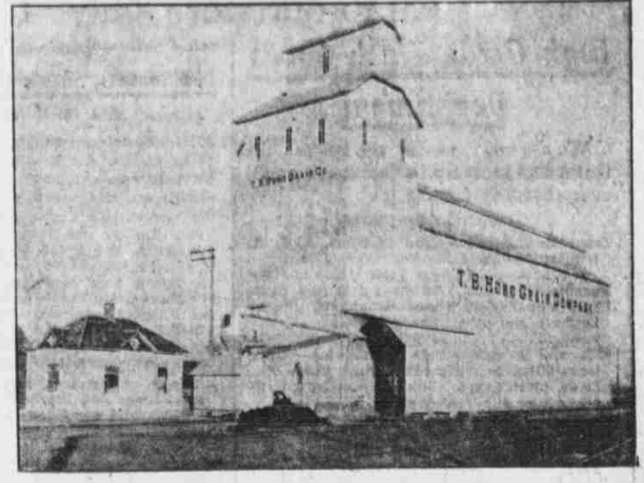
ONE OF THE GREAT GRAIN ELEVATORS AT COLUMBUS.
