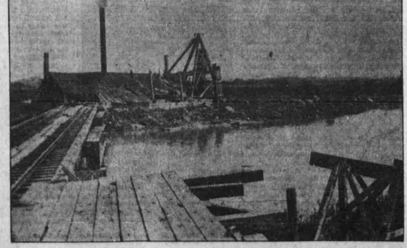
ONE OF THE SMALL DREDGES CROSSING THE ILLINOIS CENTRAL TRACKS.
