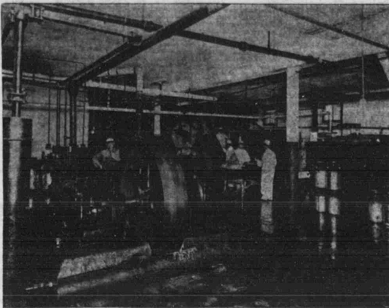
VIEW OF BASEMENT SHOWING ICE PLANT, VATS AND CHURNS.
