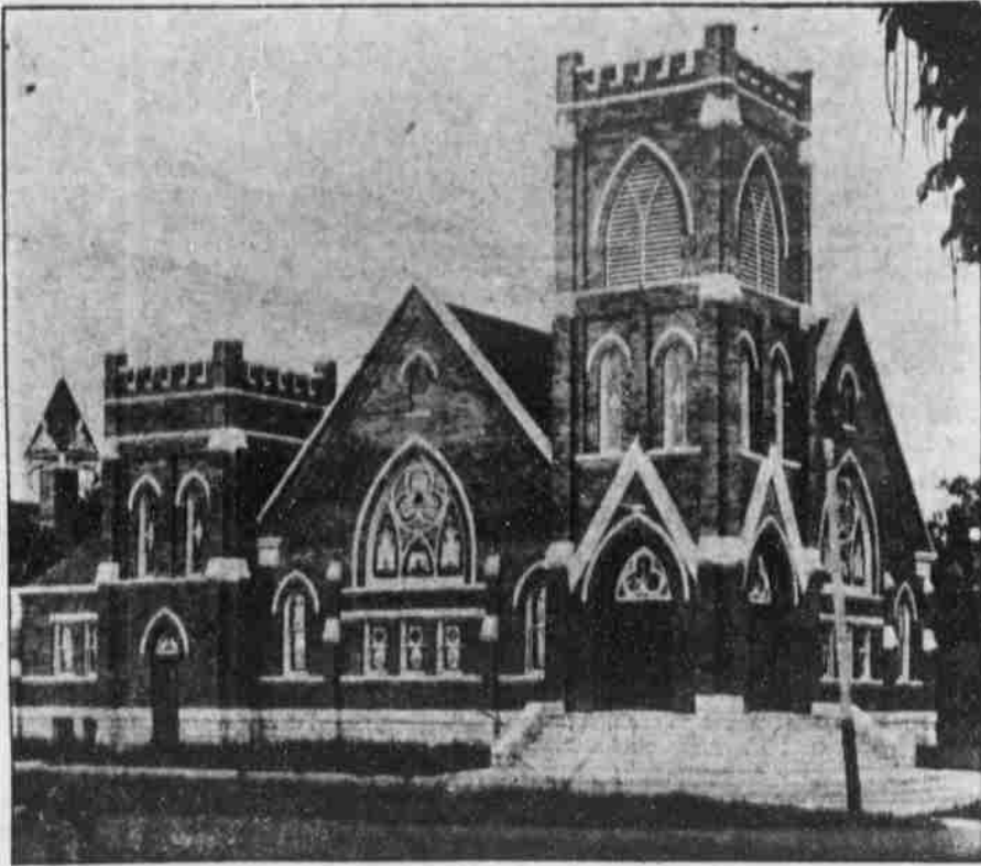
PRESBYTERIAN CHURCH AT AUBURN.
