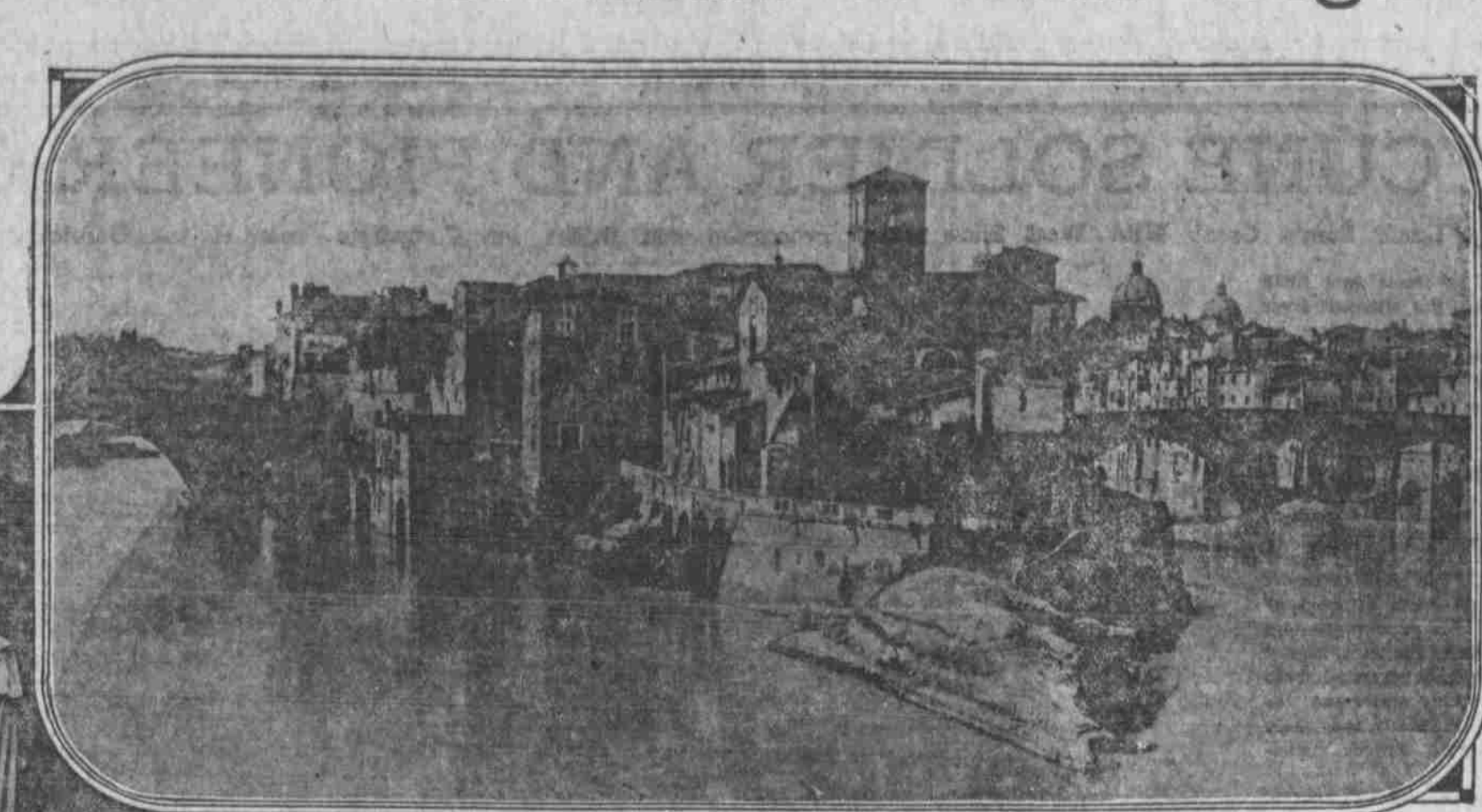
THE ISLAND OF THE TIBER WITH ITS TWO BRIDGES INTACT.
