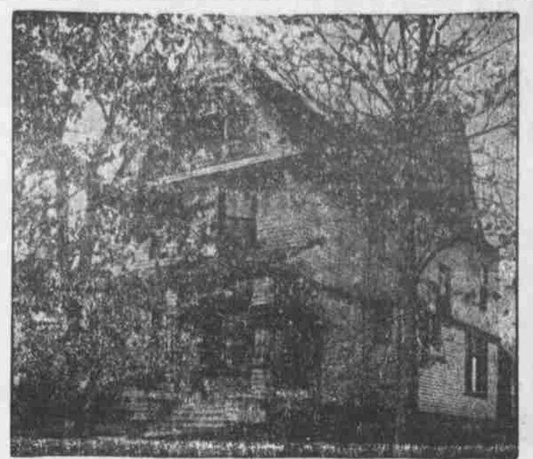
414 North 31st Street
