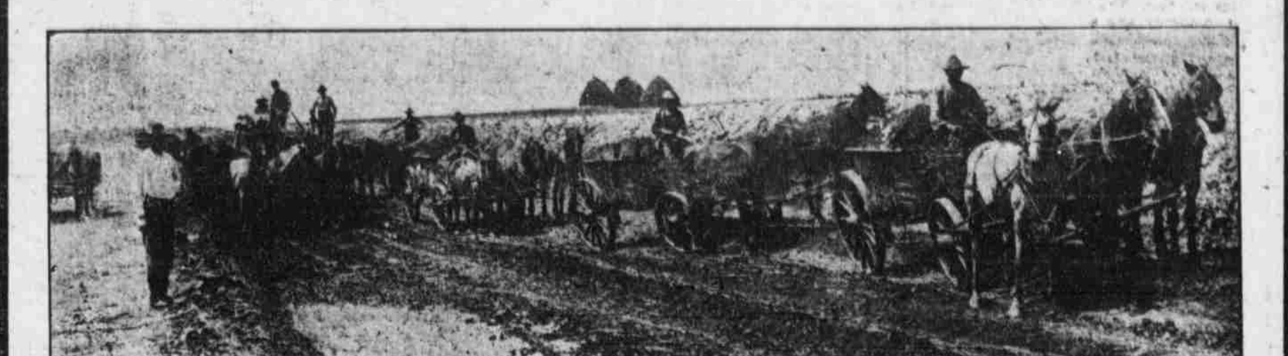
WORK ON THE ELECTRIC RAILWAY BETWEEN OMAHA AND HASTINGS.
