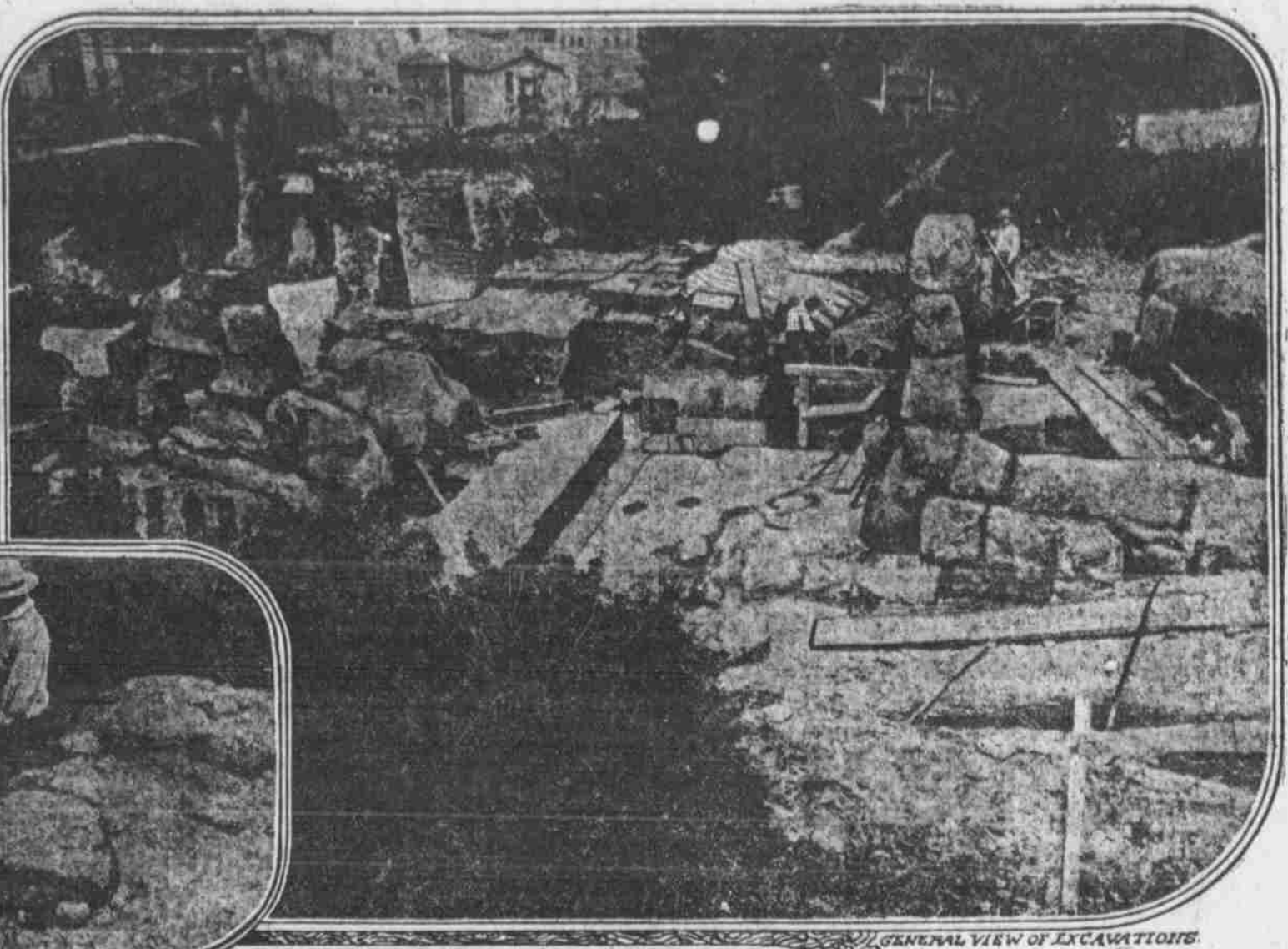
GENERAL VIEW OF EXCAVATIONS.
