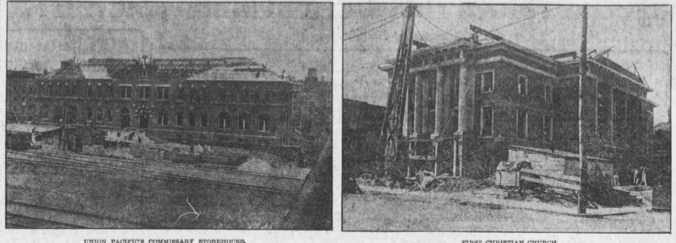
UNION PACIFIC'S COMMISSARY STOREHOUSE.
