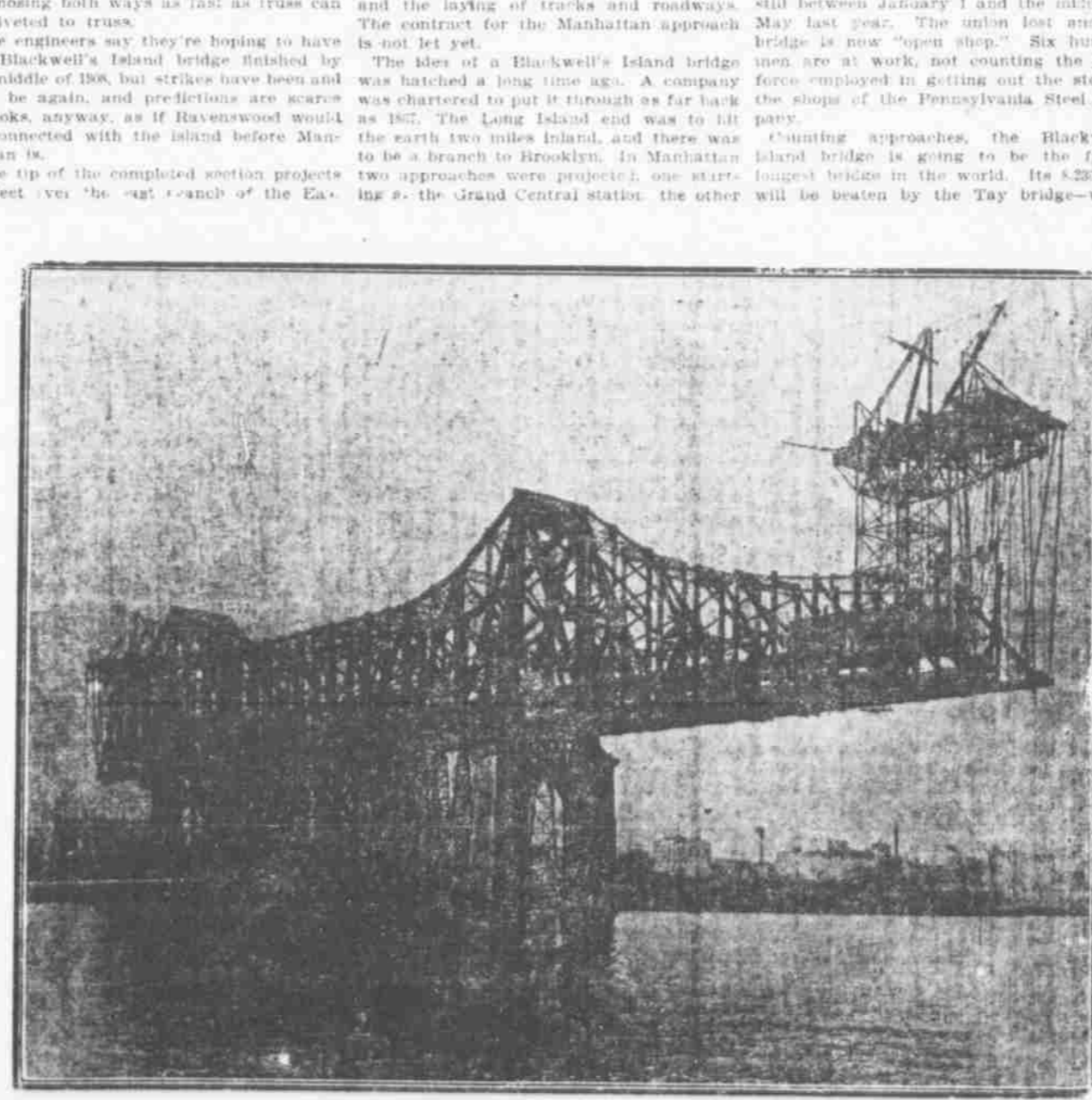
METHOD OF BUILDING THE BLACKWELL'S ISLAND CANTILEVER BRIDGE.
