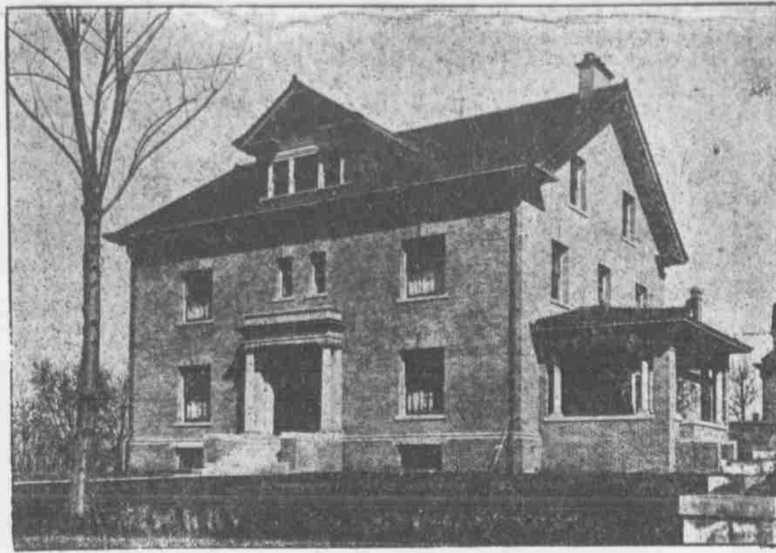
HOME OF C. D. M'LAUGHLIN, SOUTH THIRTY-EIGHTH STREET.
