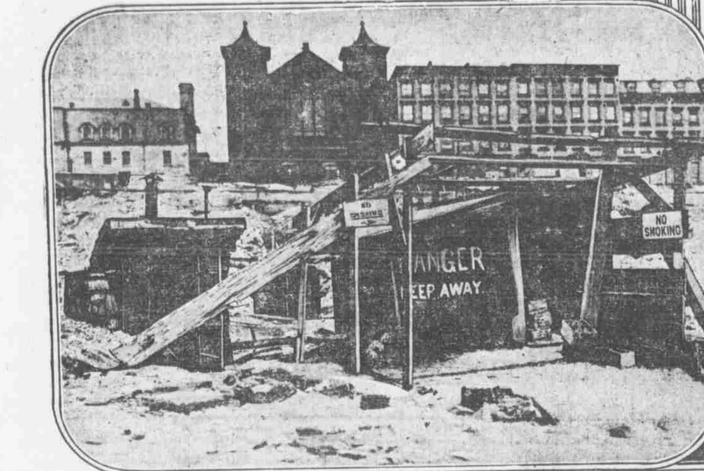
DYNAMITE EXCAVATING HOUSE PENNSYLVANIA RAILWAY TUNNEL EXCAVATION.
