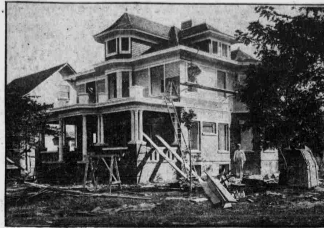
A. W. SCRIBNER'S RESIDENCE, ALMOST COMPLETED.
