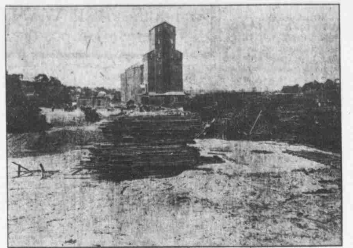
SITE OF THE NEW NYE-SCHNIIDER-POWLER ELEVATOR.
