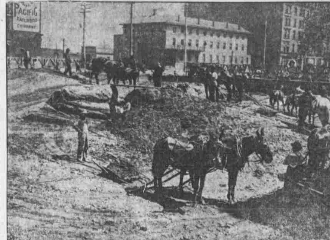
EXCAVATING FOR THE M. E. SMITH BUILDING AT NINTH AND FARNAM.
