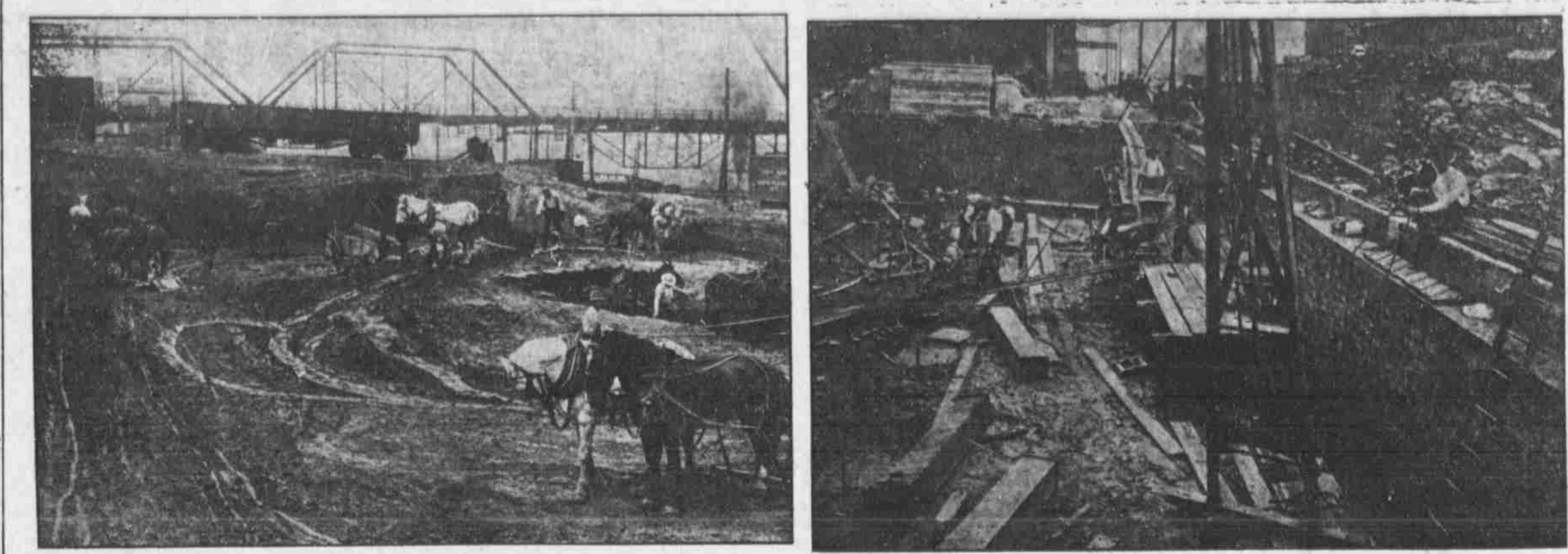
EXCAVATING FOR NEBRASKA TELEPHONE COMPANY'S WAREHOUSE AT EIGHTH AND FARNAM.
