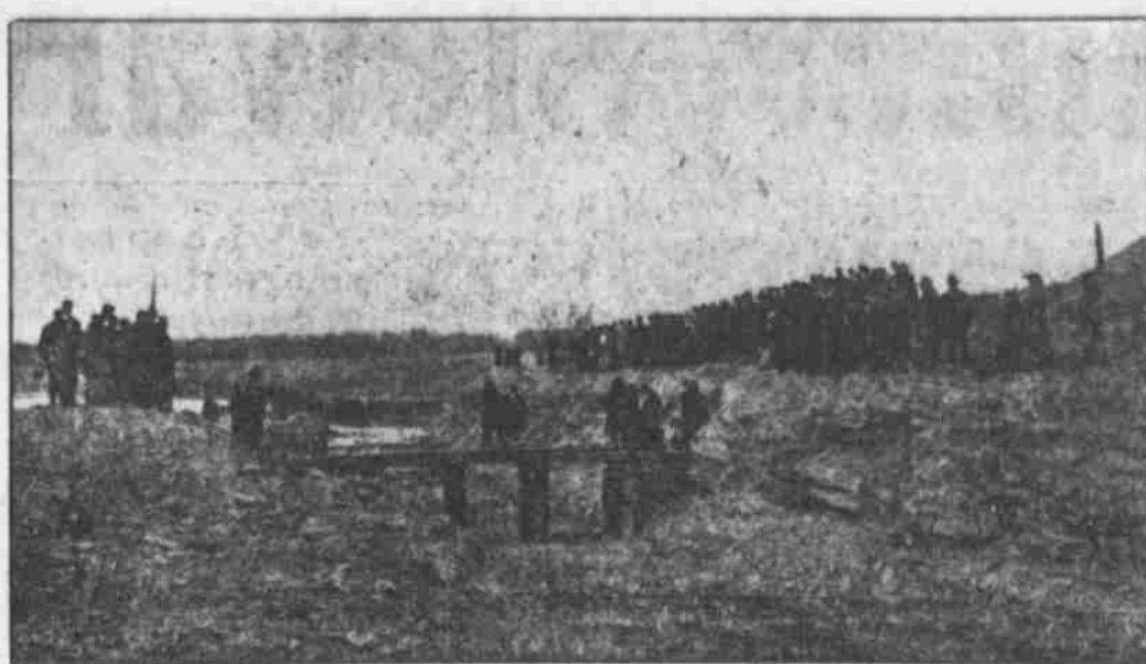
"WATER COMING" IN INTERSTATE CANAL.
