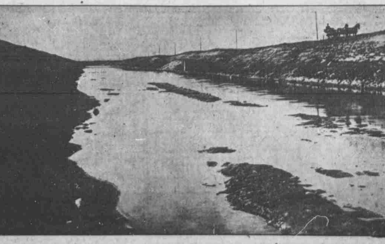
VIEW OF SECTION OF BIG ALBERTA IRRIGATING DITCH.
