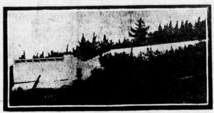
THE people of Bermuda have no mod-to meet the outlay build a "rain-catch." ern water system. Neither do wells it is a broad, whitewashed way usually supply their drinking water. Their method of supply is most primitive, but down the incline and is stored in a well-like chamber of the patience.
