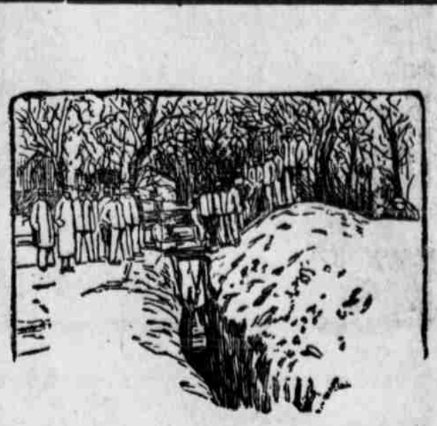
Laying Uncle Sam Pipe Line Across Neosho River
