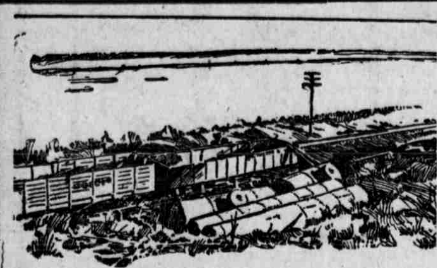
Picture of the first two carloads of pumps and boilers for the big river refinery on the banks of the Missouri by Atchison.
