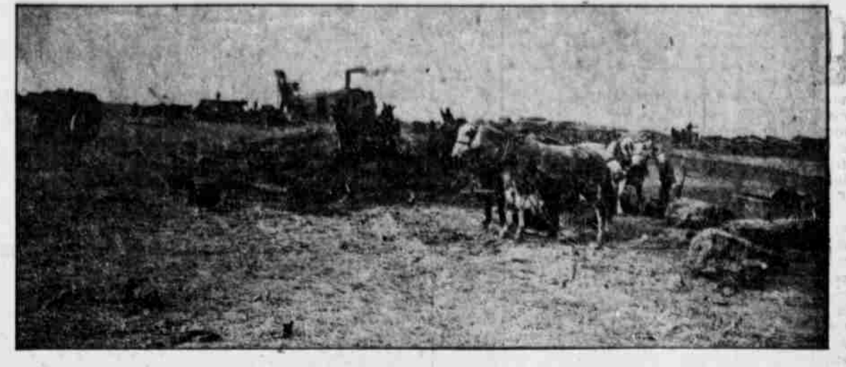
BREAKING GROUND TO LOCATE STEAM SHOVEL.
