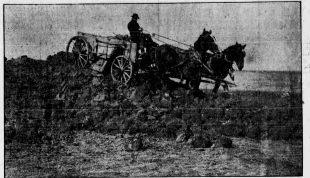
BEGINNING OF THE BIG FILL.
