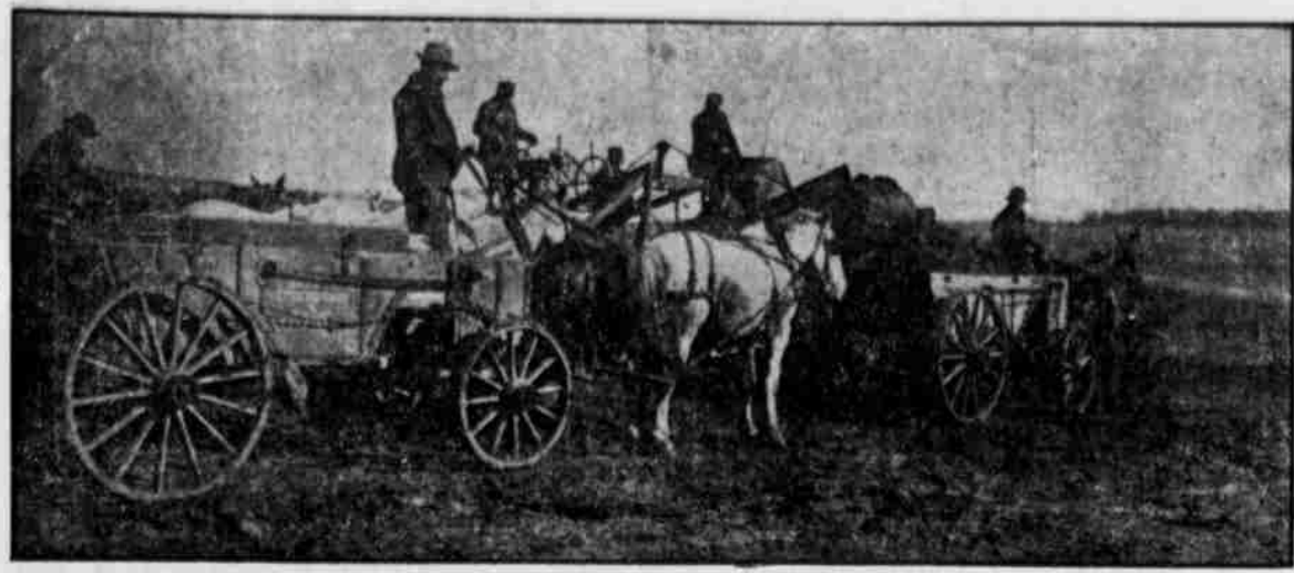
LOADING DUMP WAGONS FROM GRADER.
