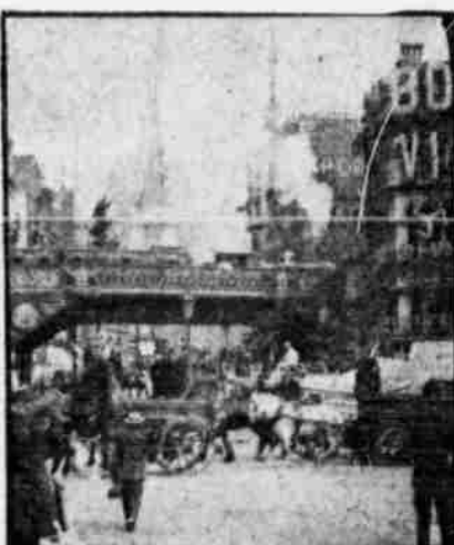
This view of Ludgate circus, in the heart of London's business district, shows the average height of buildings there. The county council building act, enforced in the city, prohibits the erection of any building over 100 feet in height. The main building may be eighty feet high, and there may be two extra stories in the roof.
