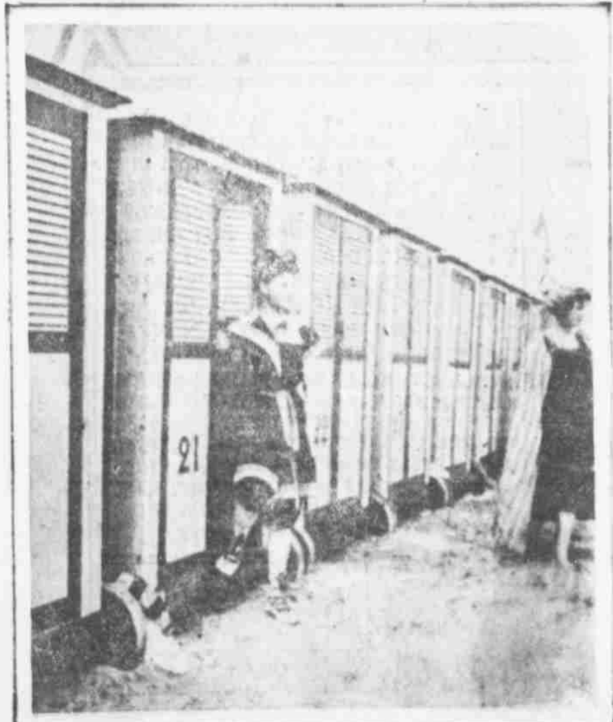
The bathhouses at French watering places are on wheels. They are rolled down beach, close to the water, so the occupants can reach the surf in a few steps.
