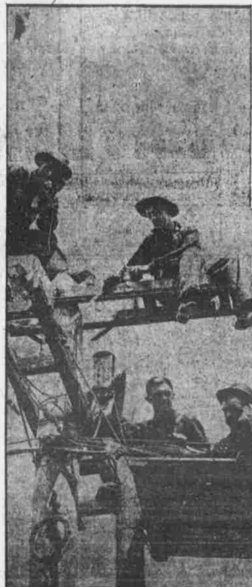
UP AMONG THE ELECTRIC WIRES.
