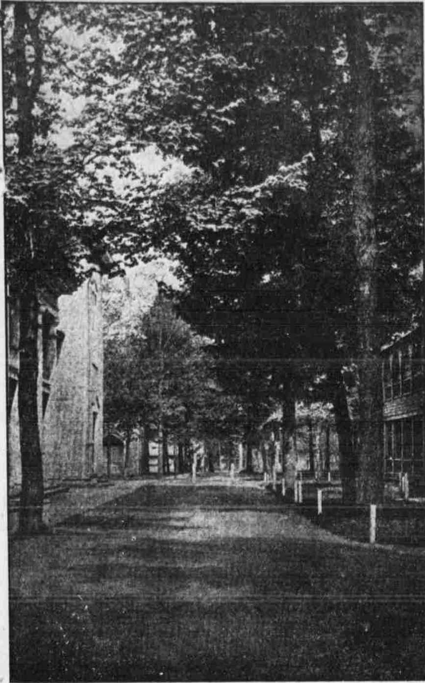
C. L. S. C. BUILDING ON LEFT—ADMINISTRATION BUILDING ON RIGHT.
