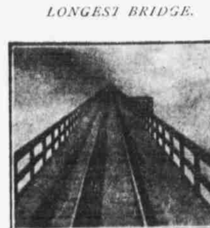
This picture represents the freestone across the Great Salt Lake. Formerly the railway crawled round the north end of the lake, but now it cuts right across it from Ogden to Lucin, thus saving 43 miles at a cost of close on $5,000,000. In building the line 22,000 miles of freestone were used, 38,250 piles were driven, each pile representing a tree cut from the forests of Oregon or Texas. If these piles had been used on an ordinary road they would cover a distance of 2,824,728.6 lineal feet, or 534,194 miles. The permanent freestone represents 11.10 miles, which is nearly all in water from 20 to 24 feet deep at the present level of the lake.
