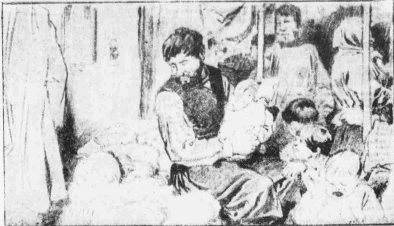
HALF A ROOM FOR A HOME: THE OTHER HALF BEHIND THE CURTAIN BELONGS TO ANOTHER FAMILY.
