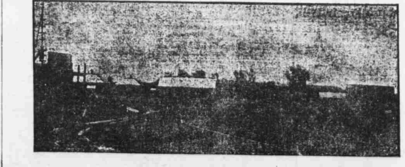
ONE CORNER OF UNCLE SAM REFINERY GROUNDS—PHOTO MAY 5.
