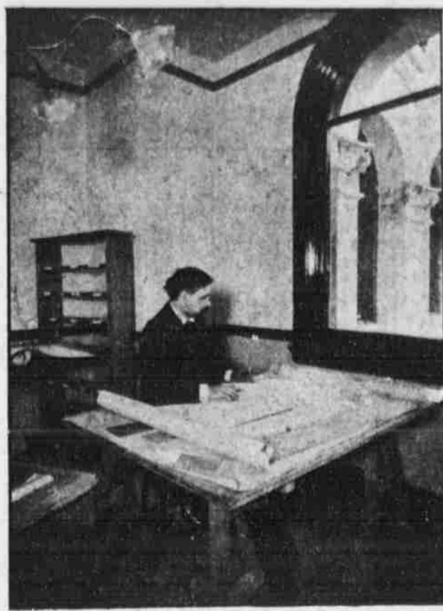
STRUCTURAL STEEL COMPUTER IN JOHN LATENSER'S OFFICE.
