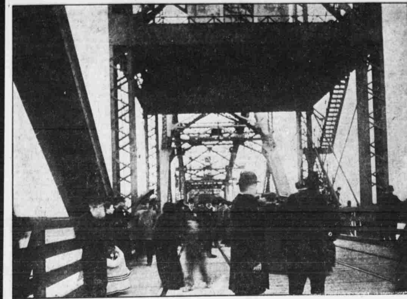
VIEW ON THE BRIDGE FROM THE WEST END.
