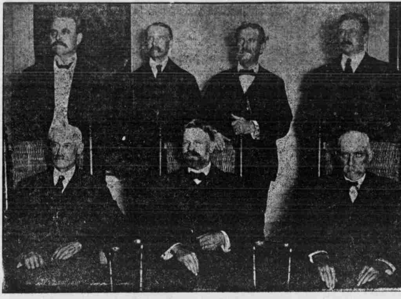
BUILDING COMMITTEE—WHICH HAD CHARGE OF ERECTION OF NEW CHURCH.
