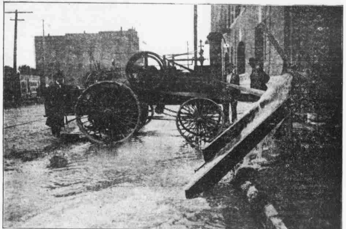
PUMPING OUT A CELLAR IN THE IMPLEMENT DISTRICT.
