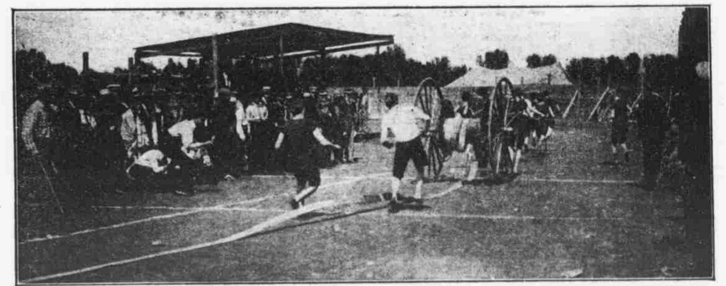
"DRY" HOSE RACE—PIPE COUPLERS READY.
