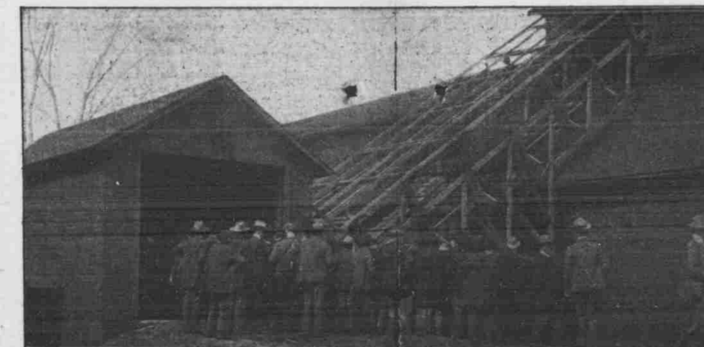
INSPECTING THE HUGE GRANARY ON BROOKMONT FARM, ODEBOLT, IA.
