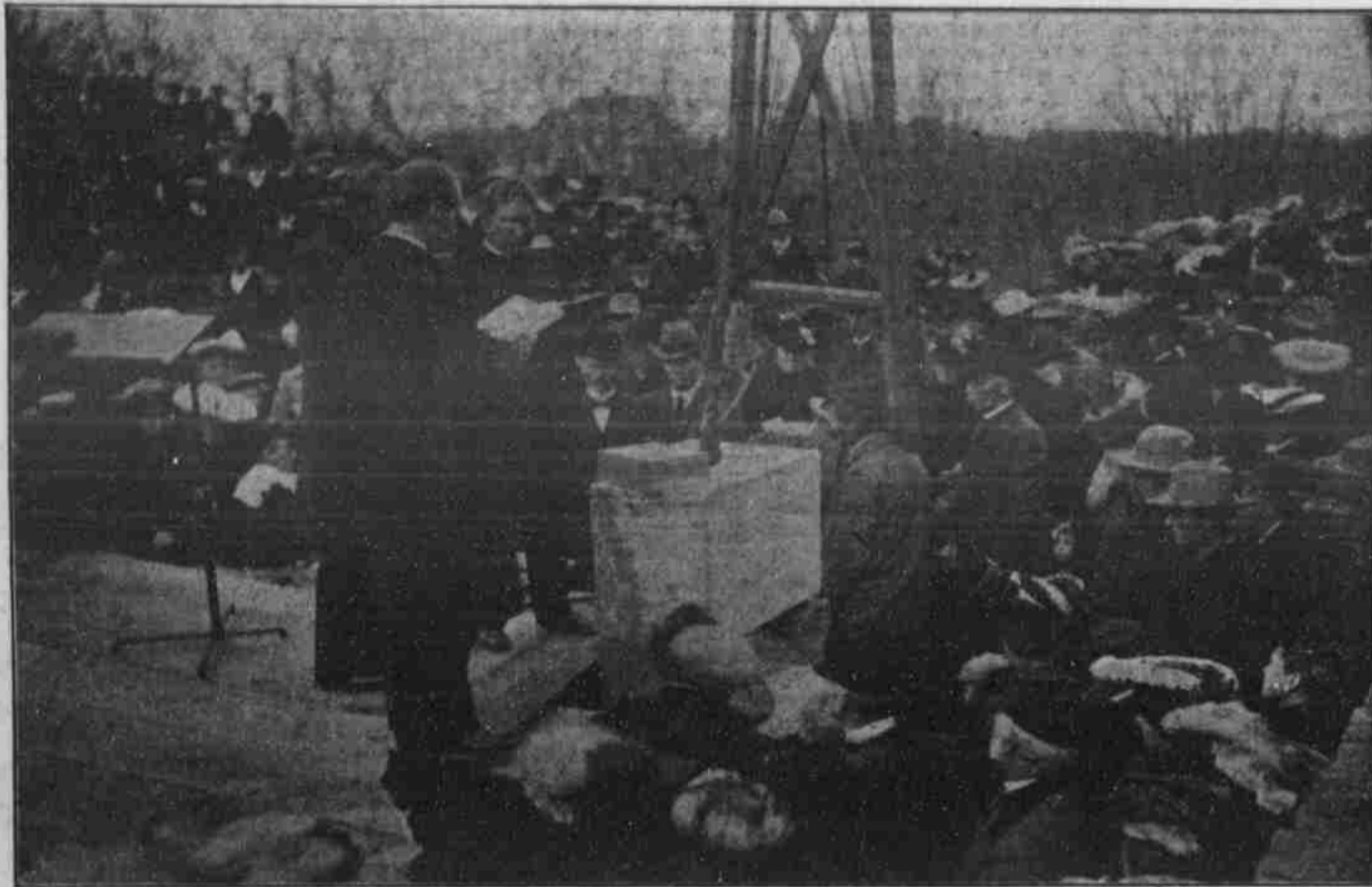
LAYING THE CORNERSTONE OF LUTHER ACADEMY AT WAHOO, Neb., ON EASTER SUNDAY AFTERNOON—Photo by N. J. Anderson, Wahoo.
