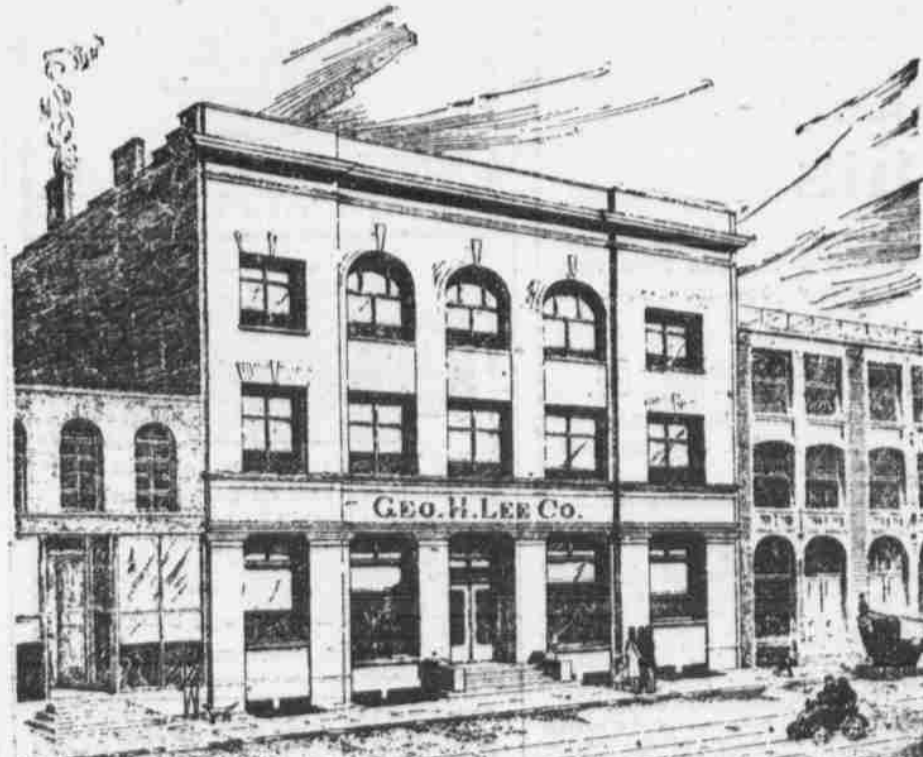
The George H. Lee company broke ground this week for their new building, 44x132, three stories high, on Harney street, between Eleventh and Twelfth. John Latenser is the architect.
