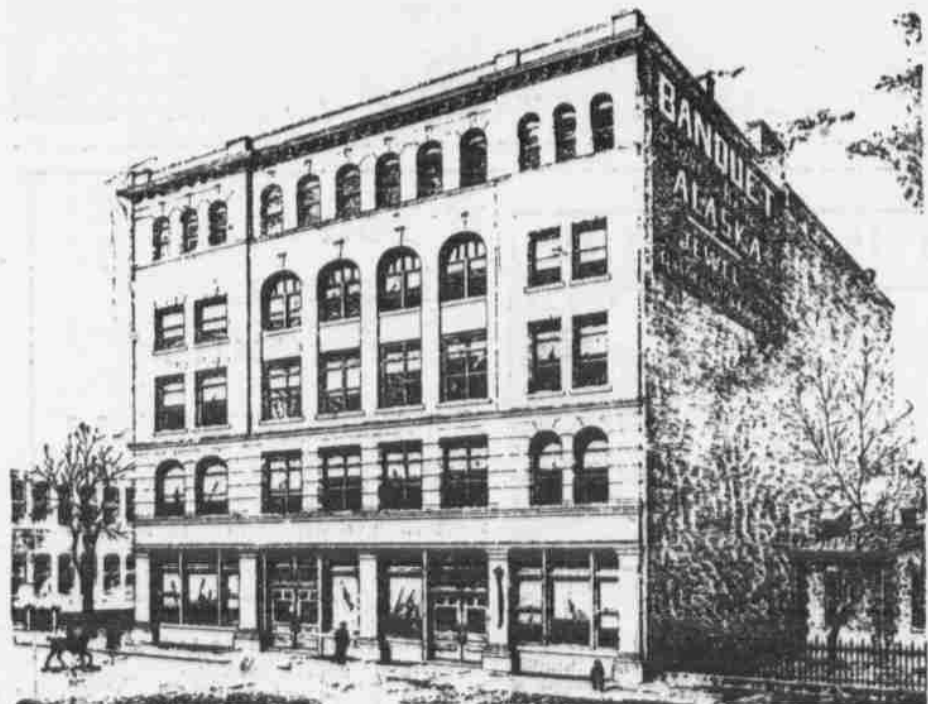
The Great Western Stove company has just completed its new building, 66x 125, five stories high, on Harney street, between Ninth and Tenth, and have moved into same. The above cut shows the structure. John Latenser was the architect.
