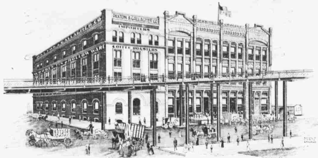
Main Offices 701 to 711 South 10th Street
