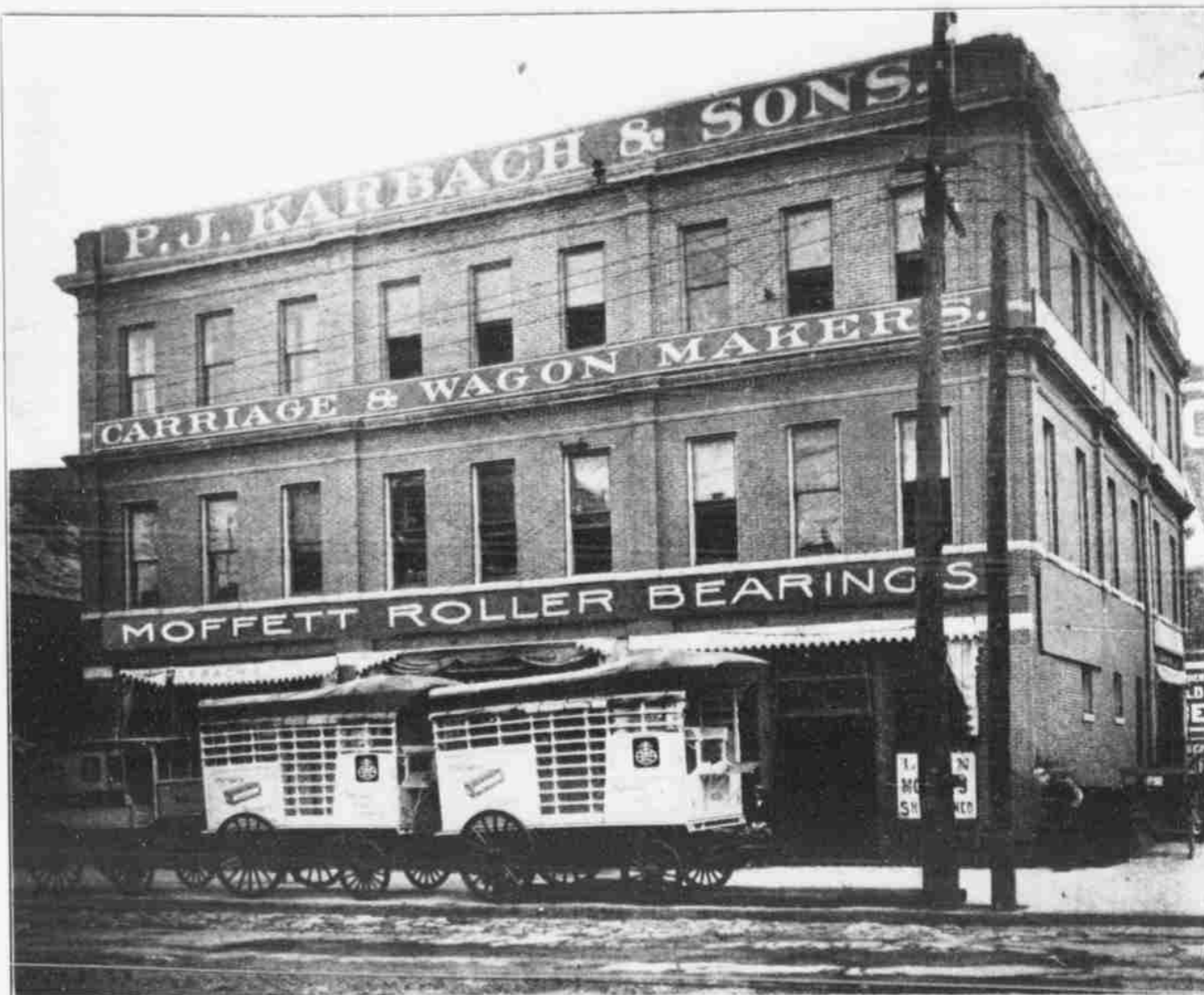
This cut is a representation of the building where 23 vehicles with MOFFETT ROLLER BEARING AXLES were built during the past season; where 437 sets of Rubber Tires were applied during the past season, besides an increase of nearly 140 per cent in our repair work. What does this mean? That we are today the foremost vehicle builders in this section of the country.
