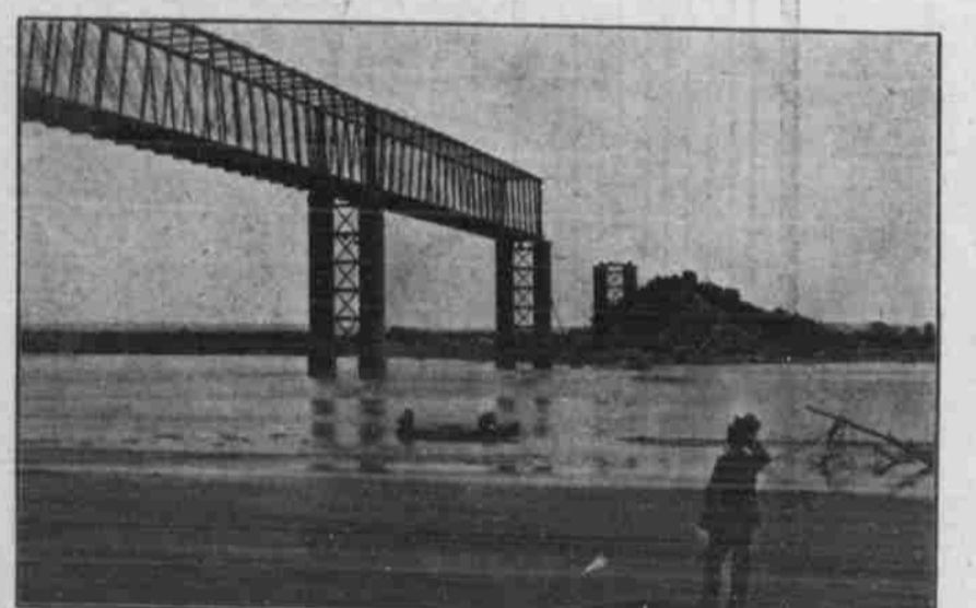
UNION PACIFIC BRIDGE AFTER THE WIND STORM OF JULY, 1877.
