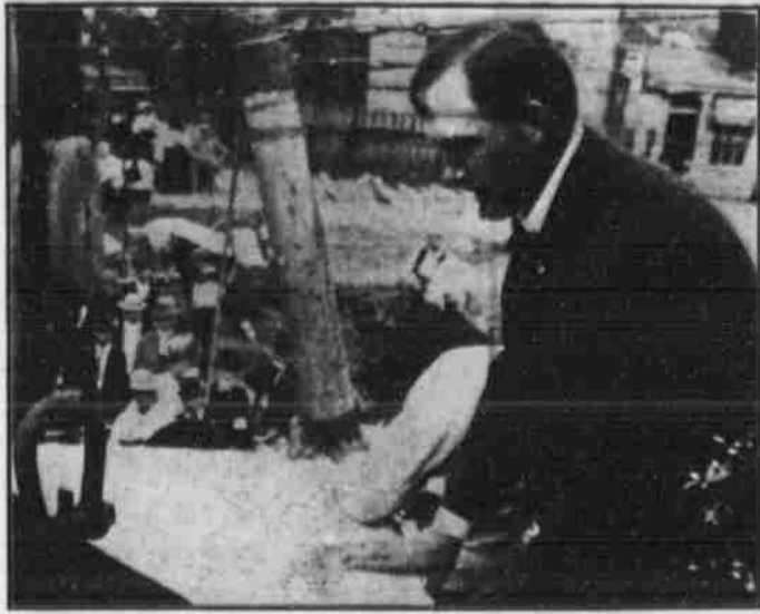
PRESIDENT SANBORN LAYING THE STONE.
