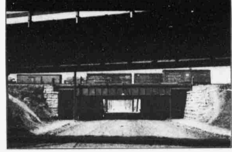
B. & M. AND U. P. CROSSING ON EIGHTH STREET.
