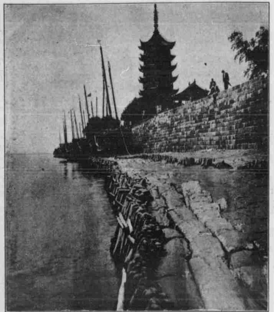
WALL AND SHIPS AT HAINUNG—THE WALL IS ONE HUNDRED MILES LONG AND KEEPS BACK THE SEA.
