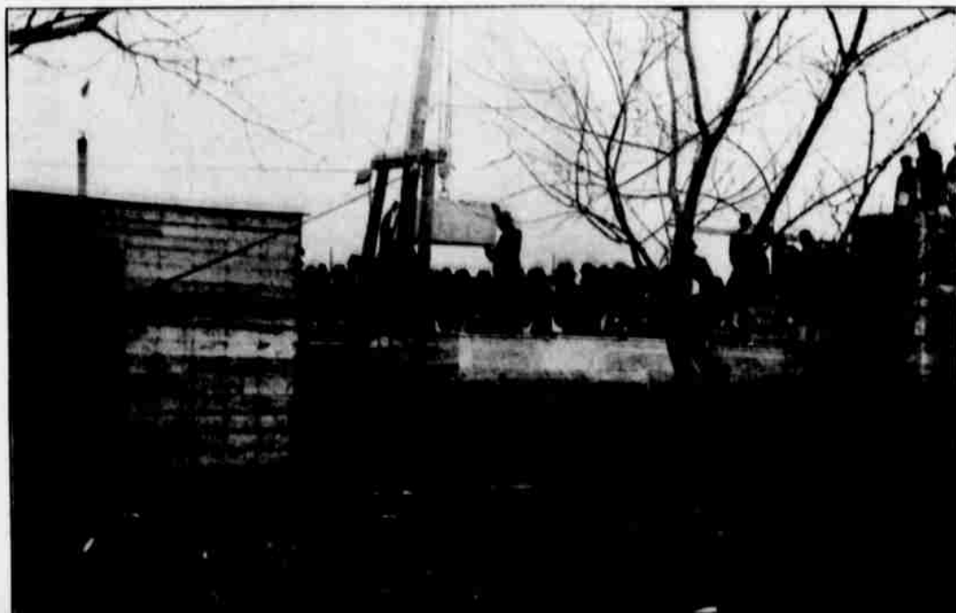
LAYING THE CORNERSTONE OF THE NEW THAYER COUNTY COURT HOUSE AT HEBRON, Neb.—LOWERING THE STONE INTO PLACE—Photo by E. A. Elder.
