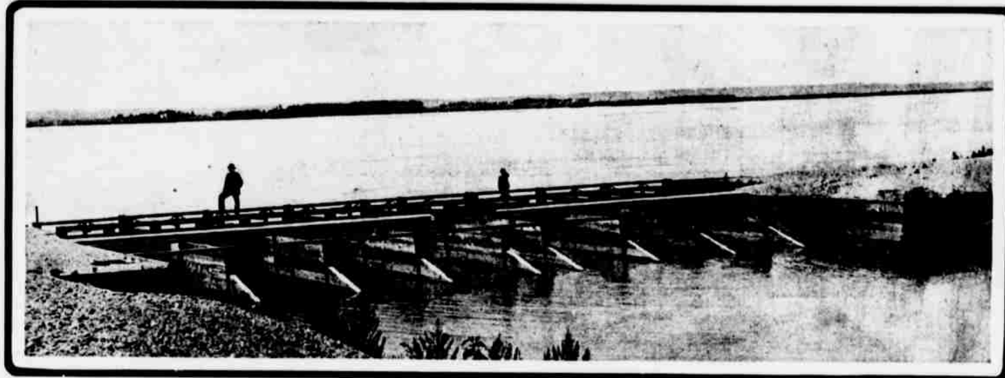
HEADGATE ON THE PLATTE RIVER, SHOWING HOW THE WATER IS DIVERTED INTO MAIN CANAL.
