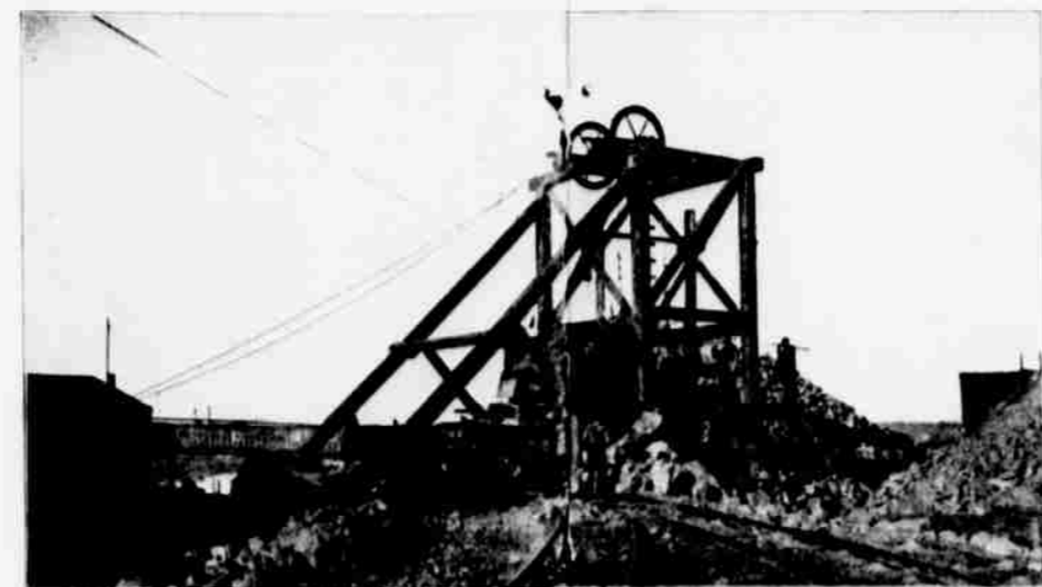
VIEW OF SHAFT ON SHERMAN TUNNEL.
