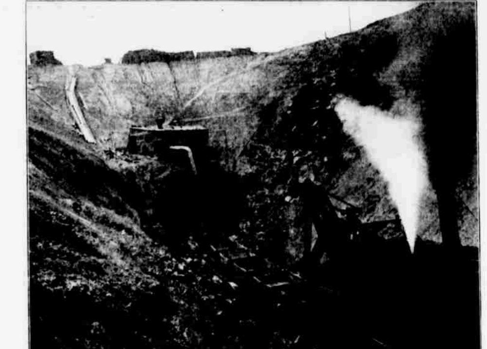
EAST ENTRANCE TO ASPEN TUNNEL—NEW LINE OF UNION PACIFIC.
