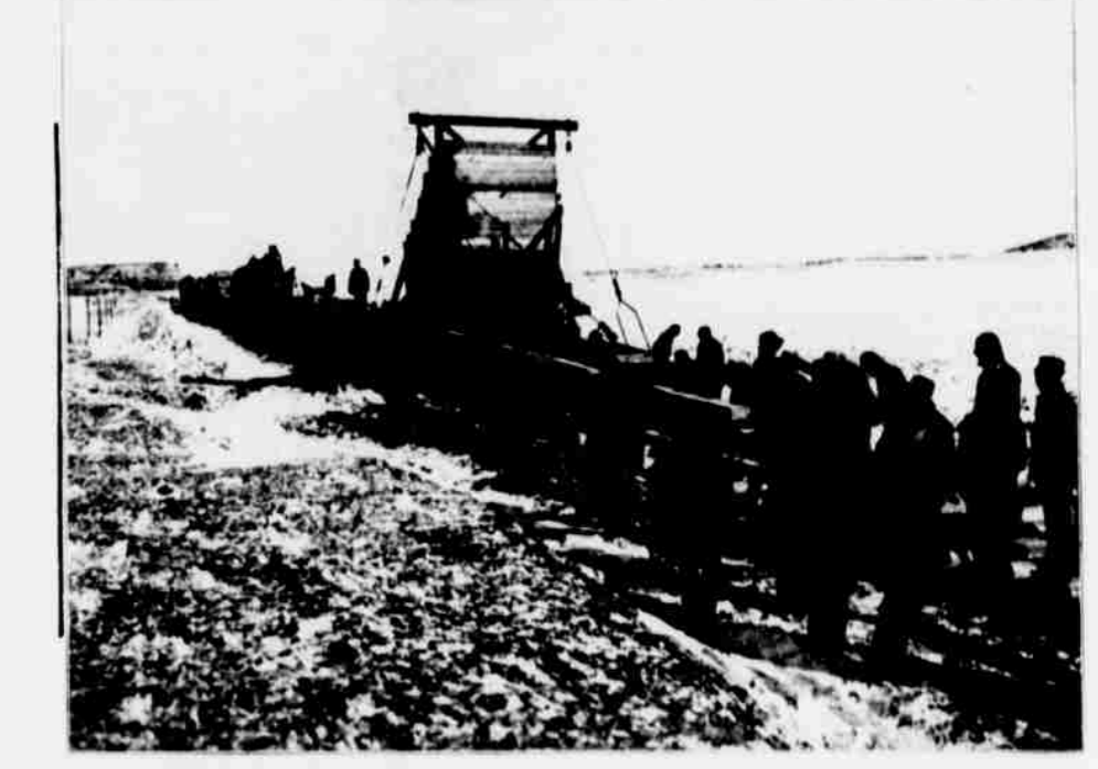
TRACK-LAYING MACHINE AT WORK ON NEW LINE OF UNION PACIFIC.
